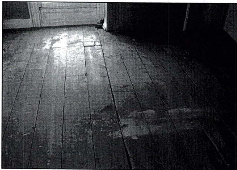
Photo 64: The wood floors of Room 202 have wood loss at the tongue and groove joints, cracks in several planks and staining.
