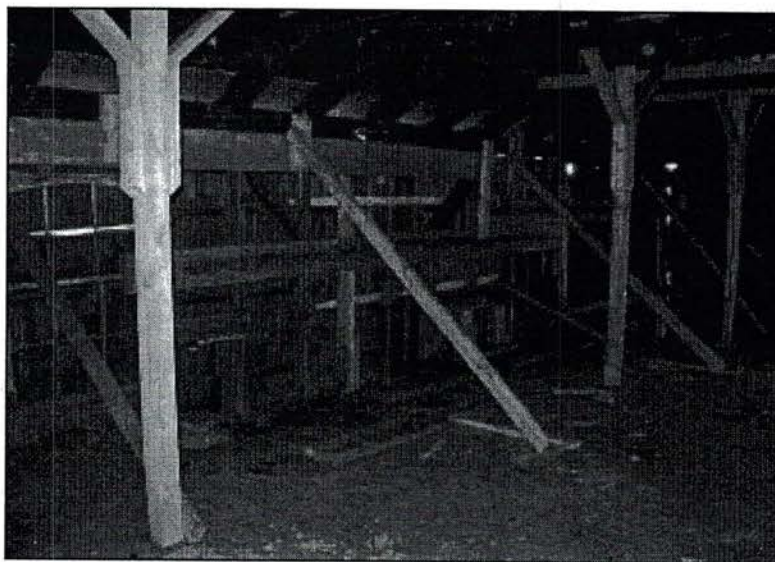
Photo 101: Second floor of the Carriage House showing temporary bracing.
