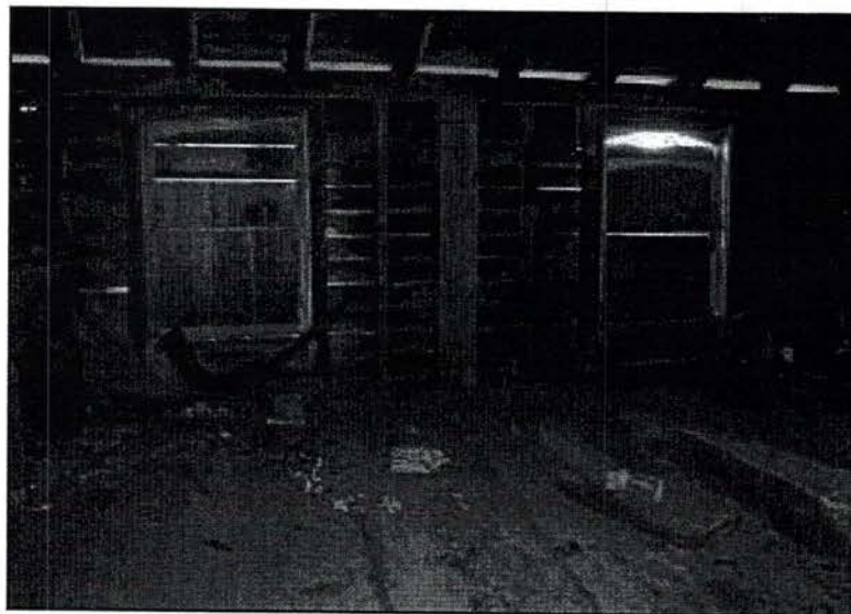
Photo 104: Southern wall of the second story of the Carriage House showing framing and partially in-tact window frames and sashes.
