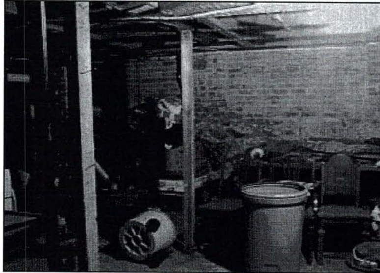
Photo 29: View looking west in Room 000 showing two of the five 2 X 4s that are being used to support the floor joists in this room.
