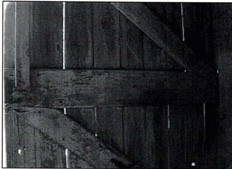
Photo 96: Detail of framing for the doors of the Carriage House.
