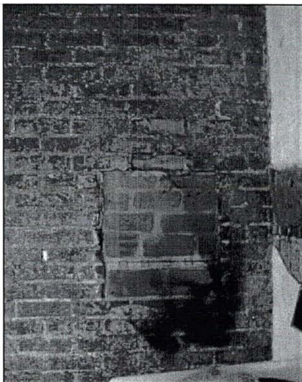
Photo 53: Possible location of a hole for a stove in Room 106.
