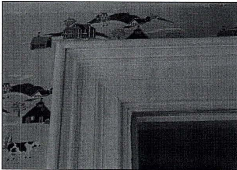
Photo 58: Detail of the door frame moldings for Room 200. These moldings are similar to the ones found on the first floor.
