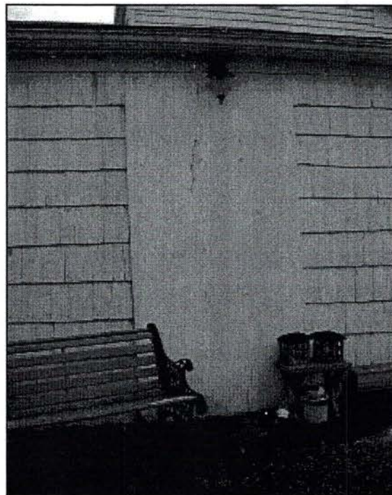
Photo 21: The door on the western elevation of the kitchen wing has been boxed-in with plywood.
