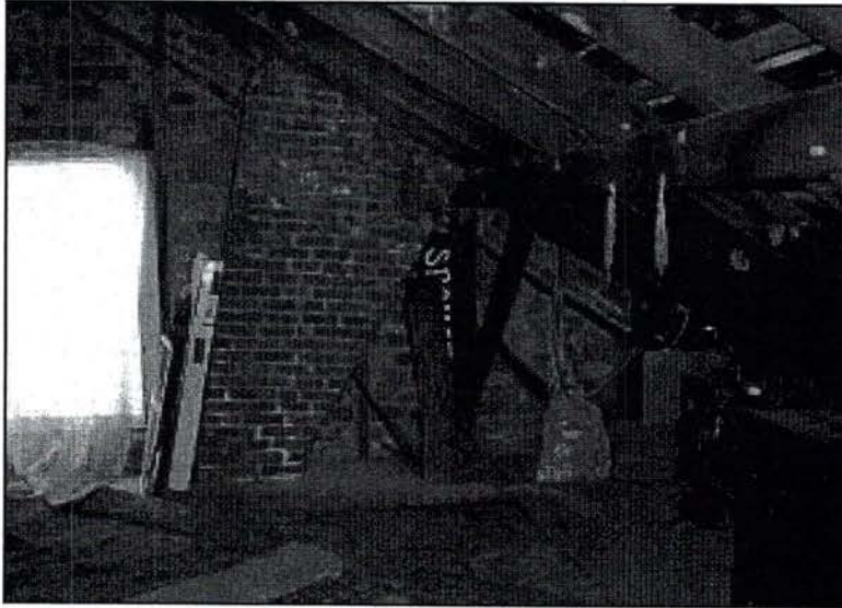
Photo 83: View looking to the northwest corner of the attic of the main section of the house showing corbeled fireplace flue, brick nogging and roof bracing. The chimney is corbeled to increase its exterior size and be more impressive.
