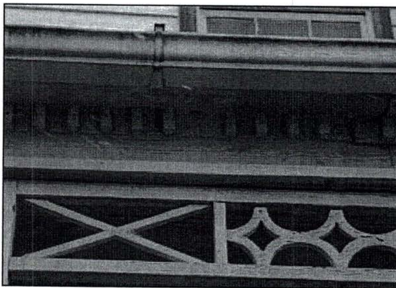
Photo 16: Detail of the decoration along the cornice of the southern porch of the rear ell. Although several dentils are missing, the majority of the decoration is intact.
