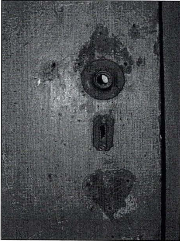
Photo 73: Ghost of Suffolk latch on the door to Room 207.
