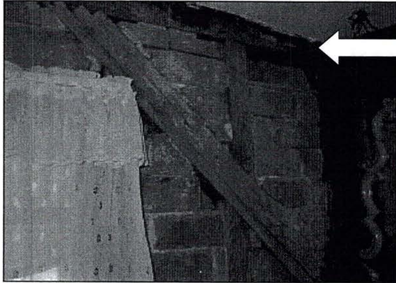
Photo 69: Plaster removed from the northern wall of Room 206 has exposed the timber framing and brick nogging of the rear ell. A recycled beam, with empty mortise joint can be seen next to the ceiling.
