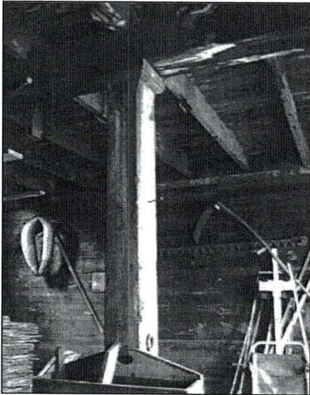
Photo 95: Chamfered post between the central bays of the Carriage House. The brick flue for the second story stove rests on this post.
