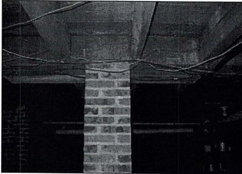
Photo 33: The brick piers supporting the girts in Room 002 were a later addition.
