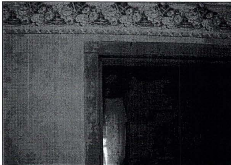
Photo 76: Door frame to Room 208. This frame is representative of the simple moldings found around the doors, windows and baseboards on the second floor of the rear ell.
