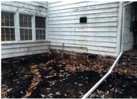
Fig. H-7 Boiler Sealed Combustion Termination
