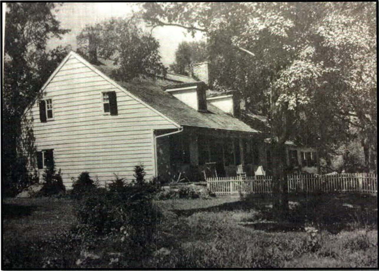
Figure 7. Van Wickle (Van Duyn) House, northwest view. This early 1930s photograph documents the dwelling's appearance after the renovations designed by architect George B. Howell, as part of which a terrace was added across the east façade and former back door on the west façade became the main entry.
