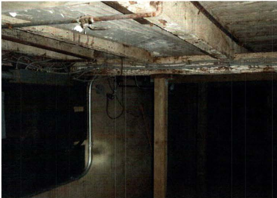
Photo T: First floor framing in Basement D
