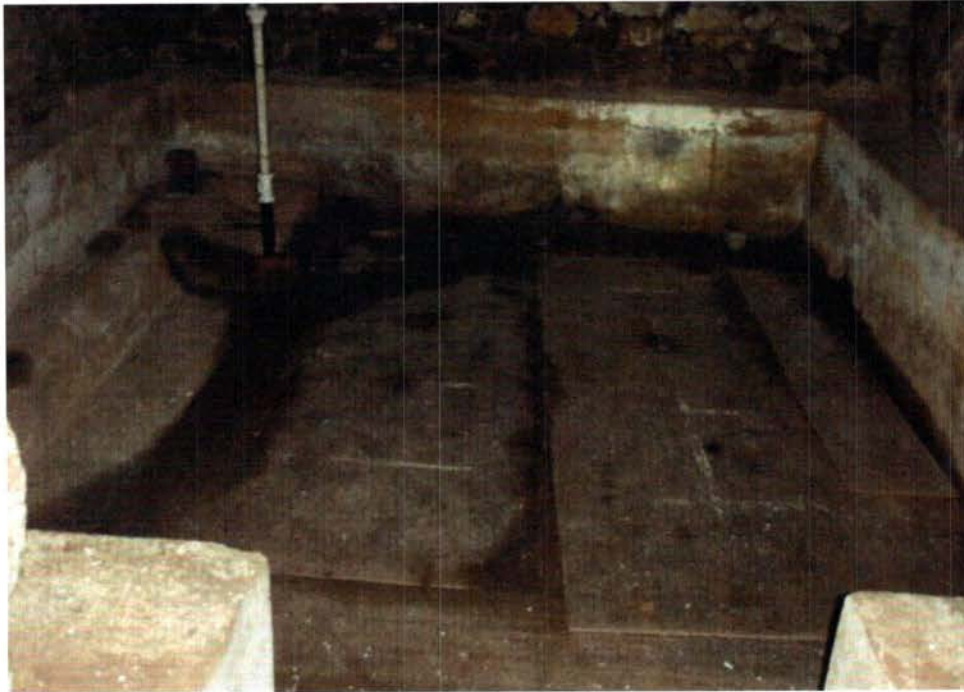
Photo O: Underpinning of Basement C
