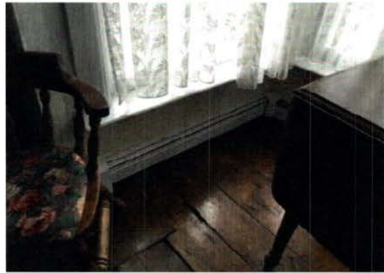
Fig. H-8 Baseboard Fin Tube Radiation (106)
