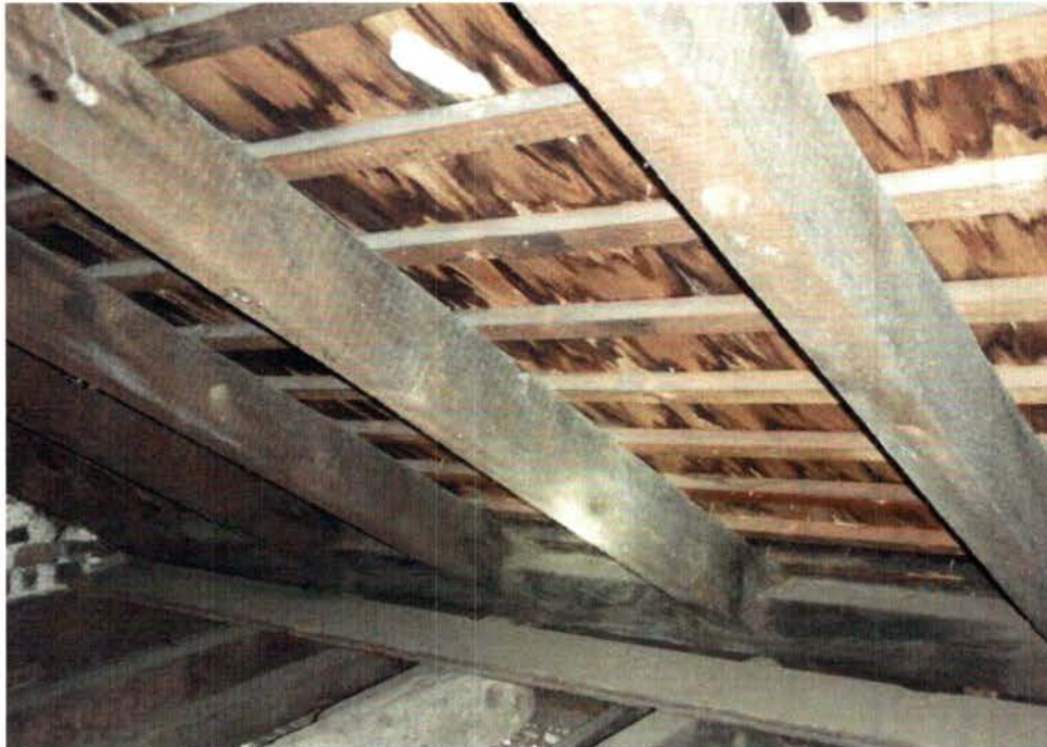
Photo L: Roof framing of the kitchen addition.
