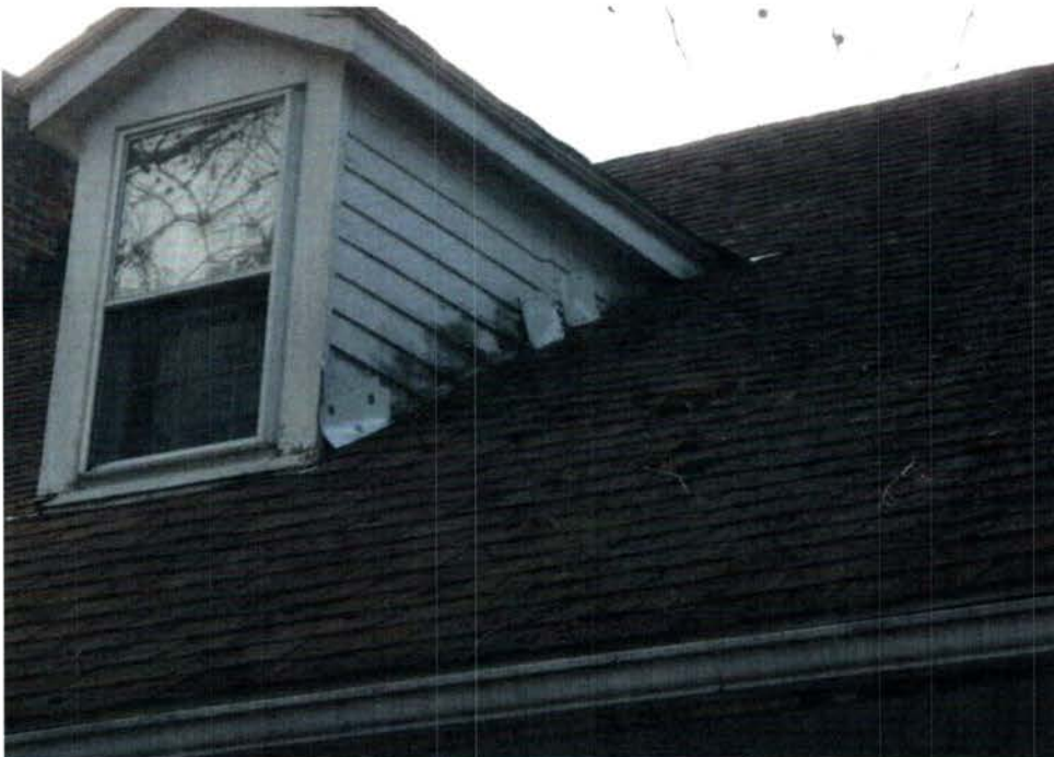
Photo C: Metal plates at south dormer on east side of original structure
