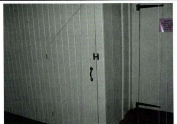
Room 107, stair enclosure with wide boards at right "Build B."
