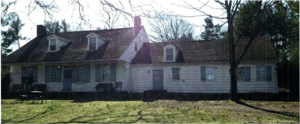
Photo 01: Main elevation with Builds A1, A2, B and C shown from left to right, as viewed looking west (from the Delaware & Raritan Canal and the Raritan River).
