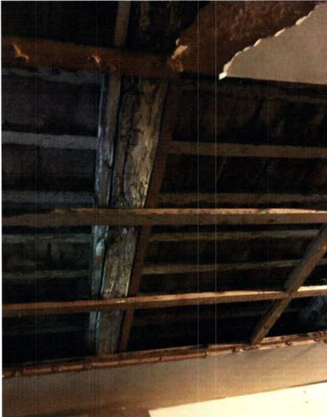
Photo I: Exposed roof framing at center addition portion of structure
