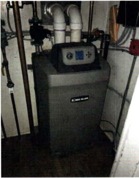
Fig. H-1 Boiler (103A)
