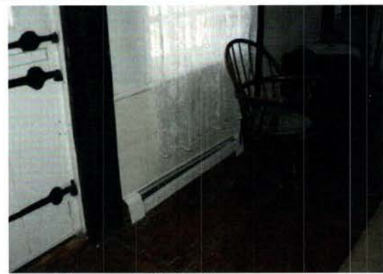
Room 103, east wall, “Build A.”
