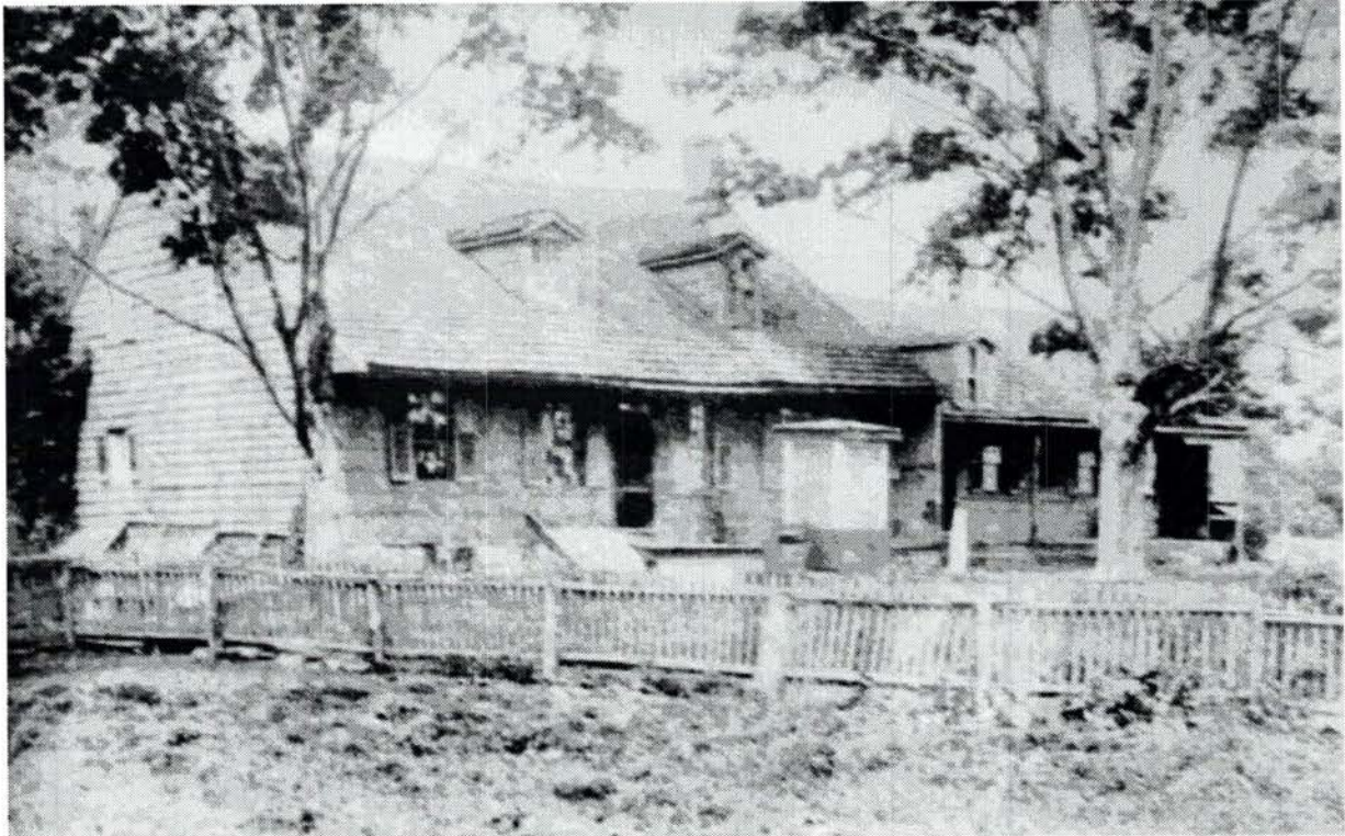
Archival photograph provided by Michael Calafati Architect, LLC, depicting east façade, apparently lacking kitchen addition associated with "Build C."
