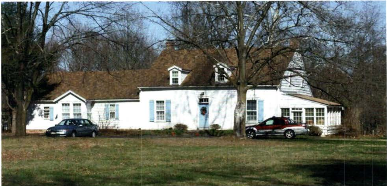
Photo 18: Overall view of the house's west elevation, looking east in the direction of the Delaware & Raritan Canal and Raritan River, with Builds C, B, A2, A1 and D shown from left to right. The current main entrance, Door A, is at the center of the main block and would be adapted to provide ADA/Barrier-Free access. Build D, the hothouse, would be demolished.
