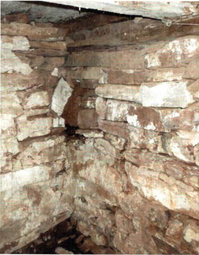
Photo N: Southwest corner of Basement A foundation wall
