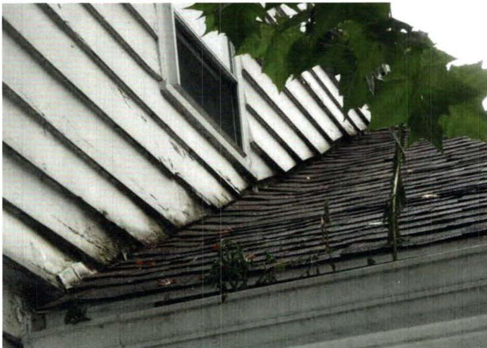
Photo D: East side of center addition roof adjacent to the original structure.
