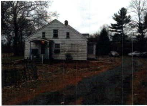
Figure E-1 Service Entrance (North Elevation)
