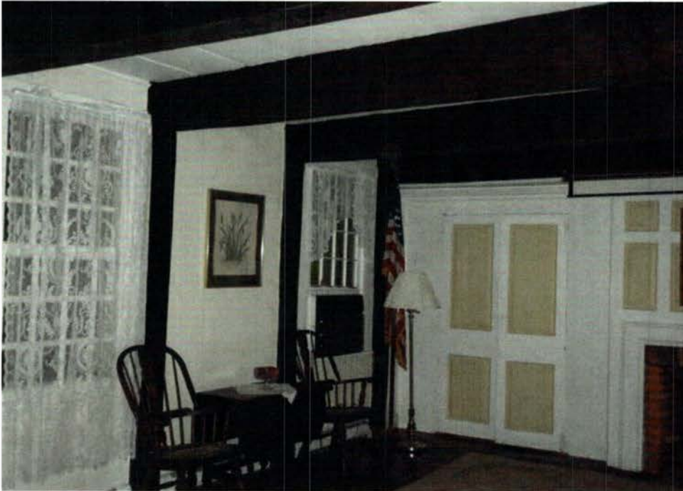
Photo M: Second floor framing in Living Room (103)
