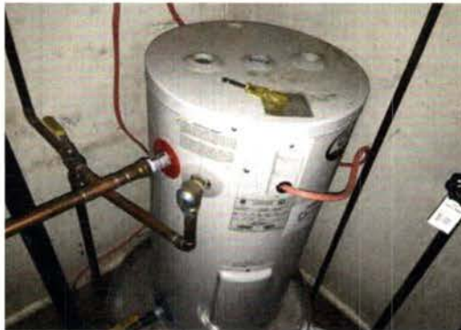
Fig. P-3- Electric Water Heater (103A)
