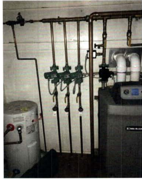
Fig. H-2 Boiler, Piping & Pumps (103A)
