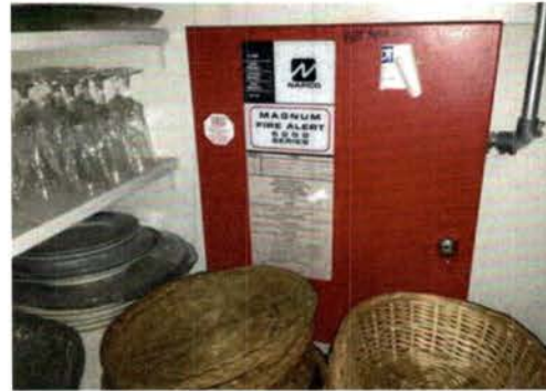
Figure E-14 Fire Alarm Panel (108A)
