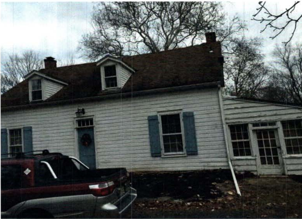
Fig. P-9- Exterior Roof Leader – Roof Leaders were previously piped underground.
