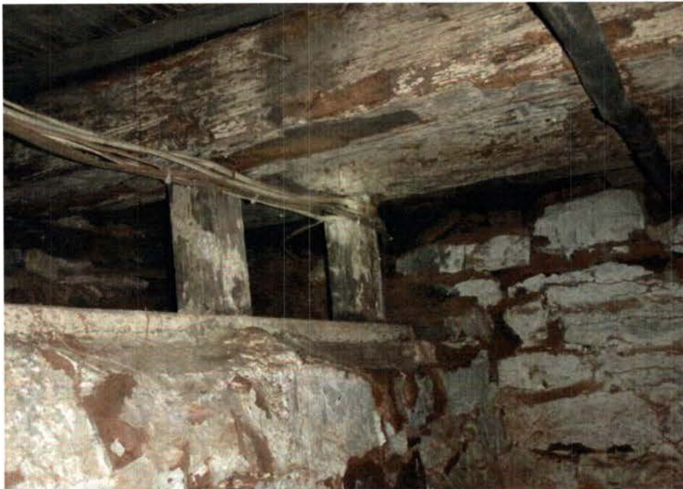
Photo P: Low wall at east side of Basement C
