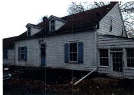
Figure E-10 Exterior Lightng (Over Door and at Corner)
