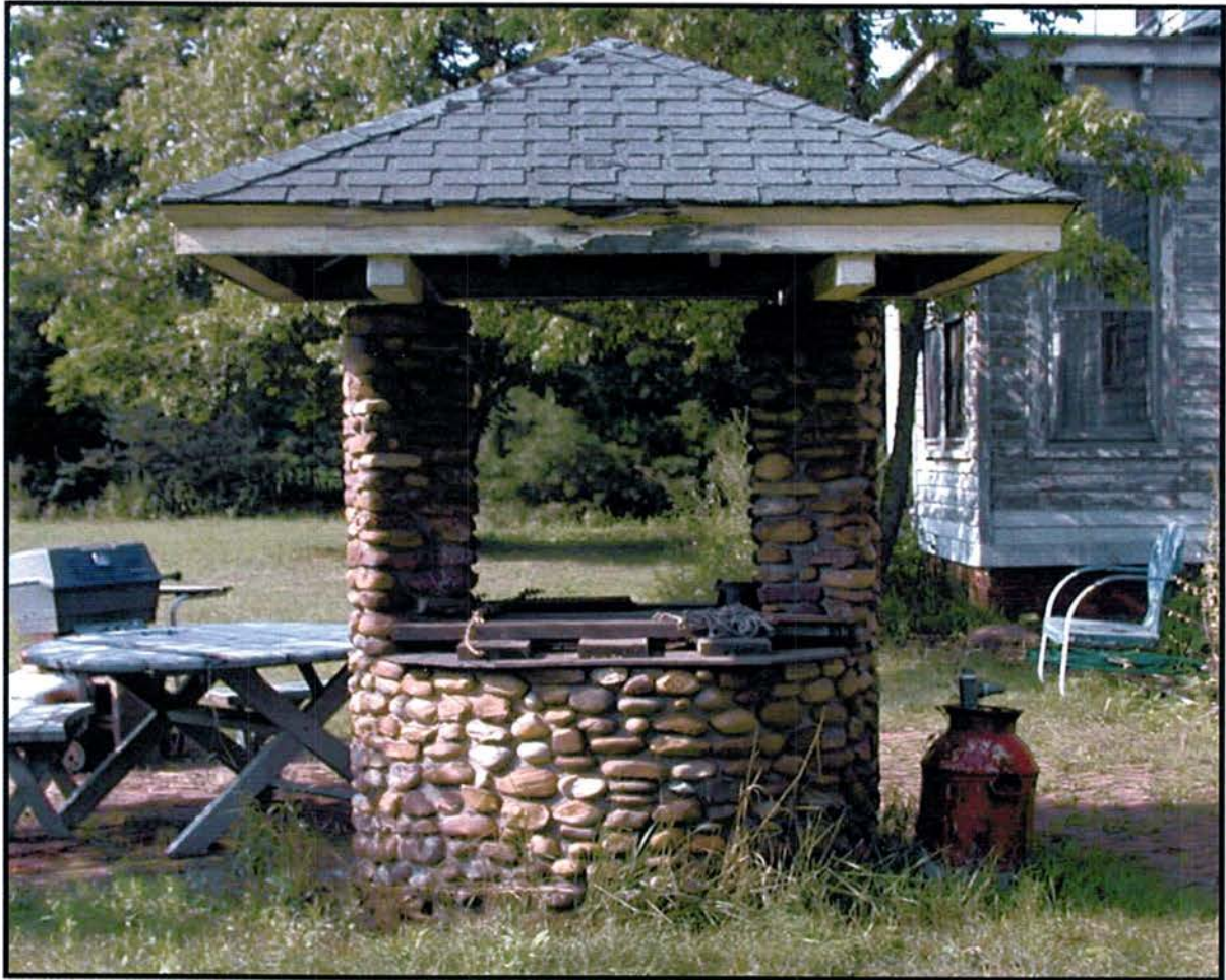
Close-up view of covered well.
