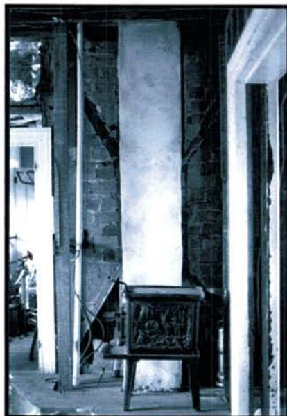
Four views of the front and rear parlors, showing the partially-stripped plaster walls and the process of renovation undertaken during the 1990s.
