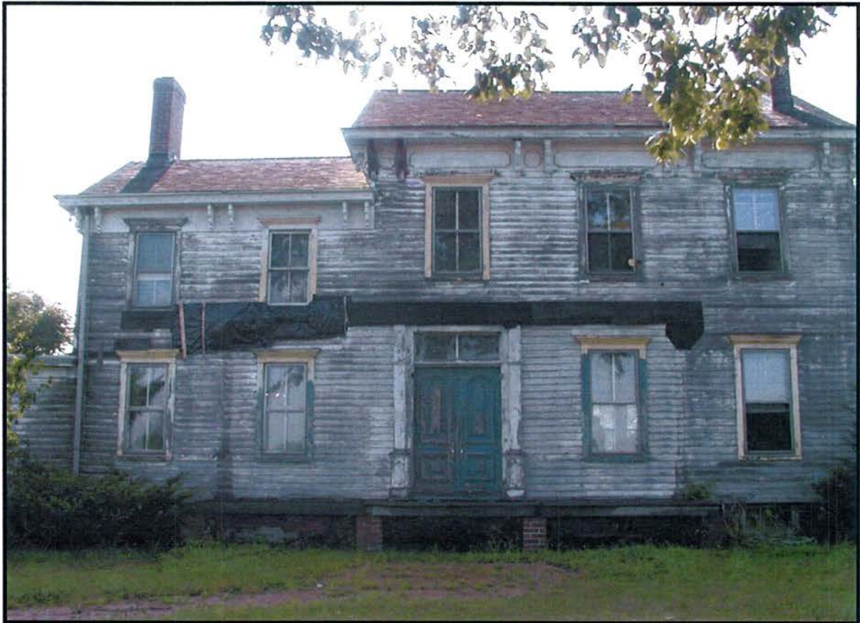
West facade view, showing area covered by former porch.
