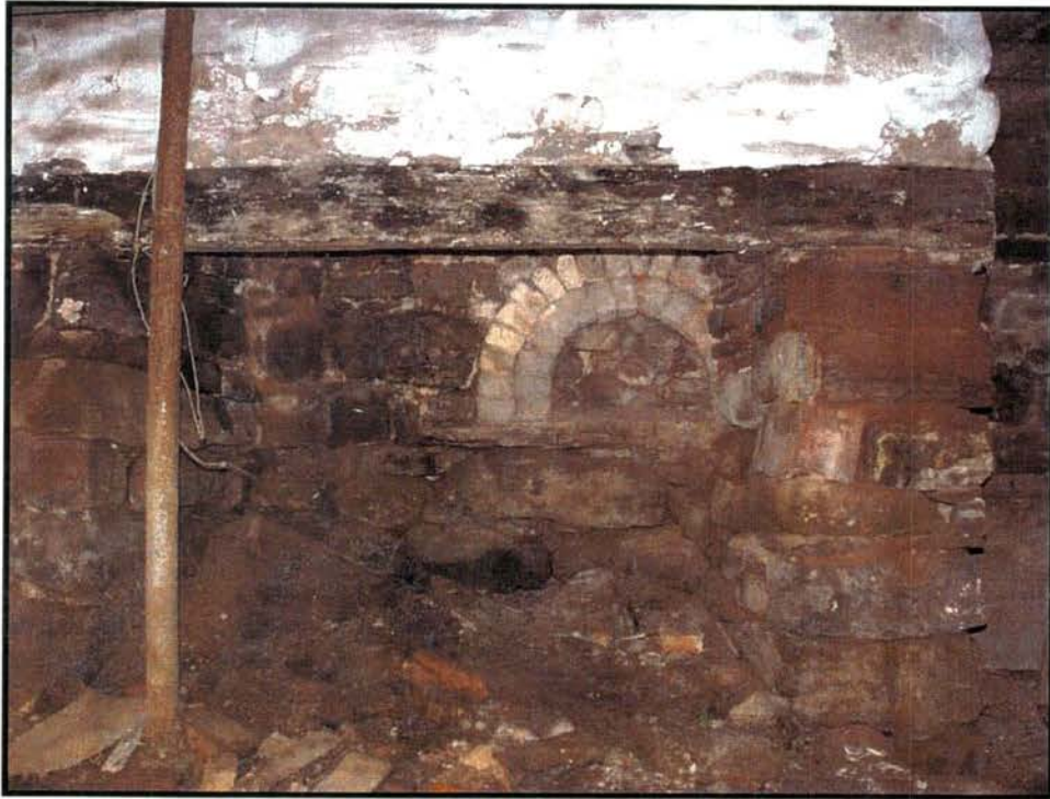
Plate 1. View looking southwest showing the side walls, wood lintel and chimney massing for the fireplace in the basement of the southern section of the house; the blocked brick-arched opening in the rear of the fireplace gave access to the bake oven (Photographer: Vincent Maresca, November 2000) [HRI neg. # 00050/D1:9].
