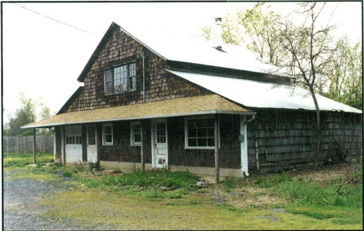
Carriage barn from the northeast. The building shows Dutch influences, but was probably constructed in the late 19th or early 20th century.
