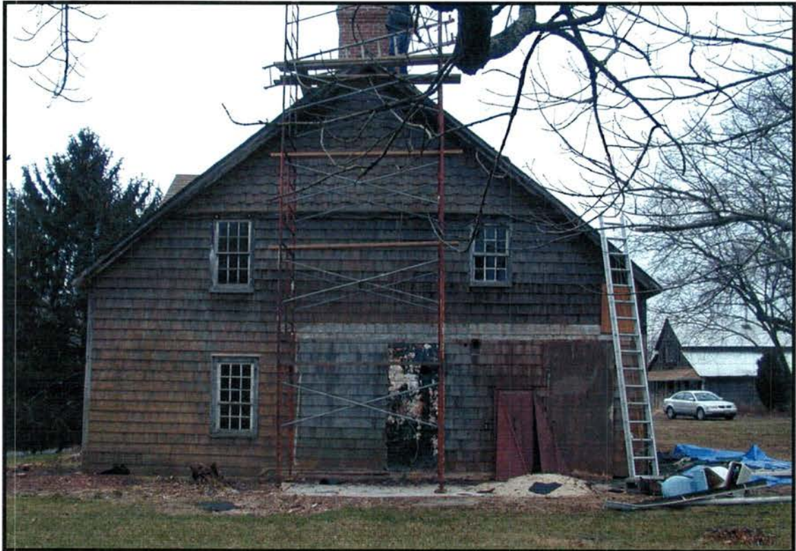
Similar view of north facade in late fall 2000, without the lean-to. Note the exposed chimney at the lower right, and former door.
