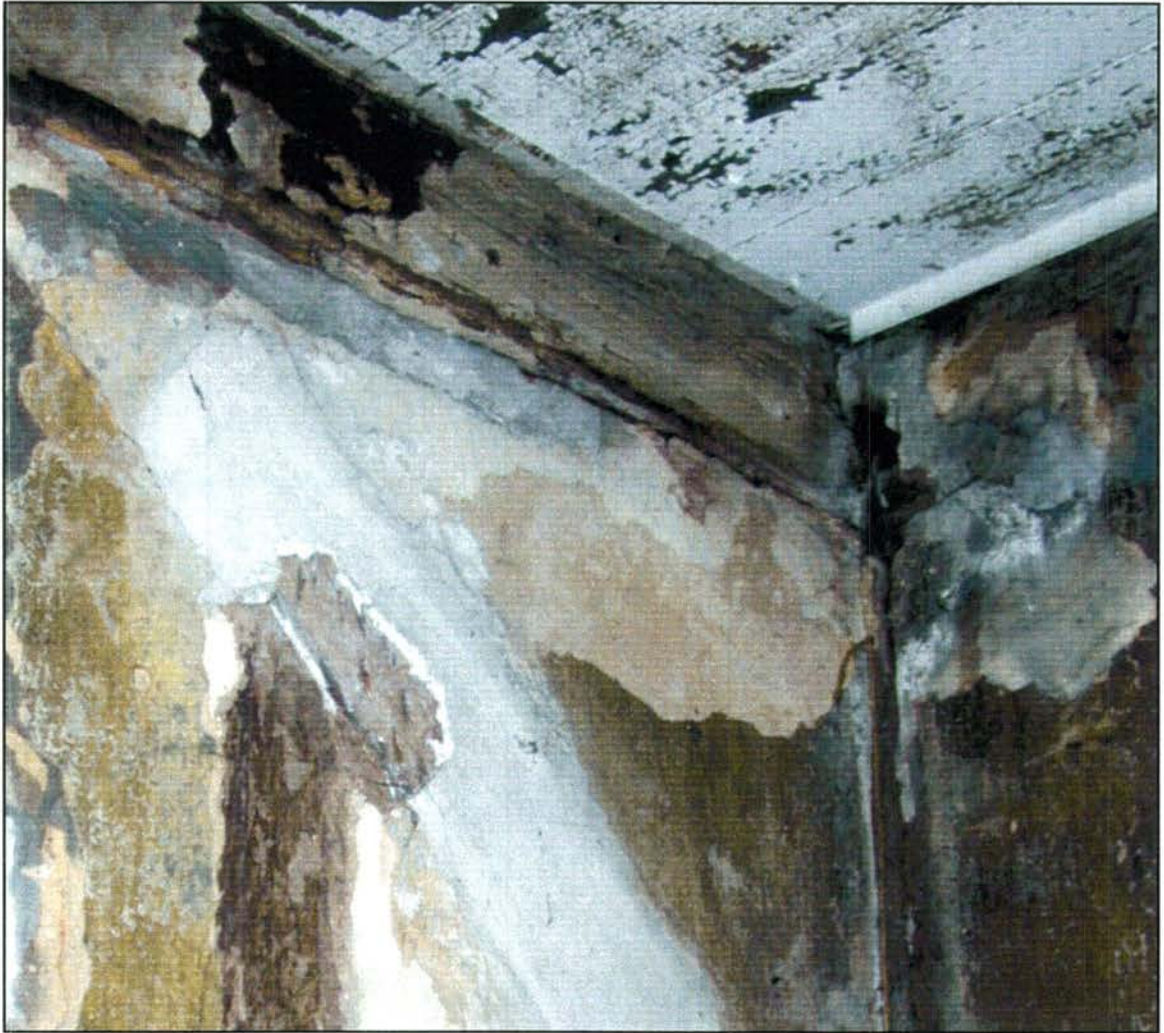
Room 102, close up view of corner, south and west walls. The joint reveals the new post, corner brace and anchor bent of the 1805 build.
