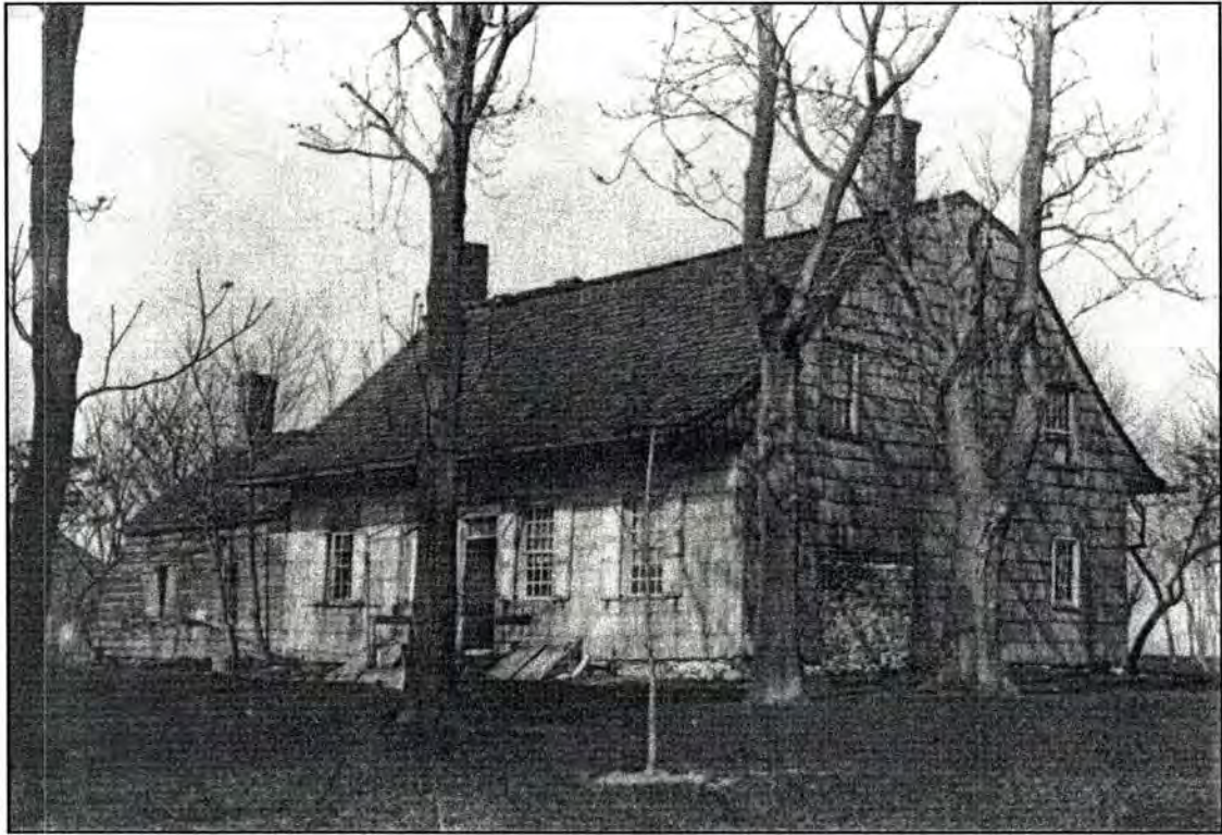
Nicholas Schenk house, Carnarsie, Brooklyn, circa 1775. With its spring eaves and gambrel roof, this is the classic "Dutch Colonial" dwelling in the common imagination.
