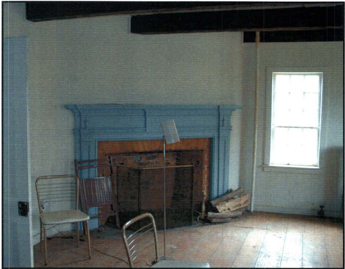
Room 105, Northeast parlor or dining room.
