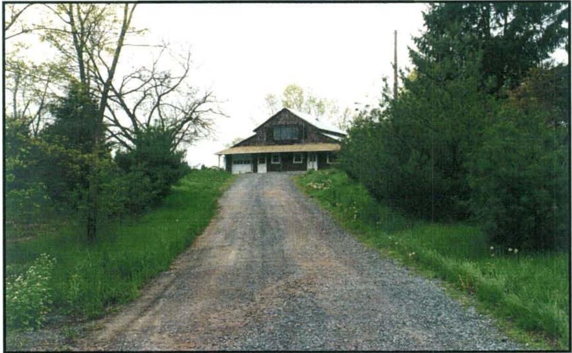
Approach drive to Wyckoff-Garretson site, following approximate path of historic access to farmstead. The carriage barn is at the top of the drive.
