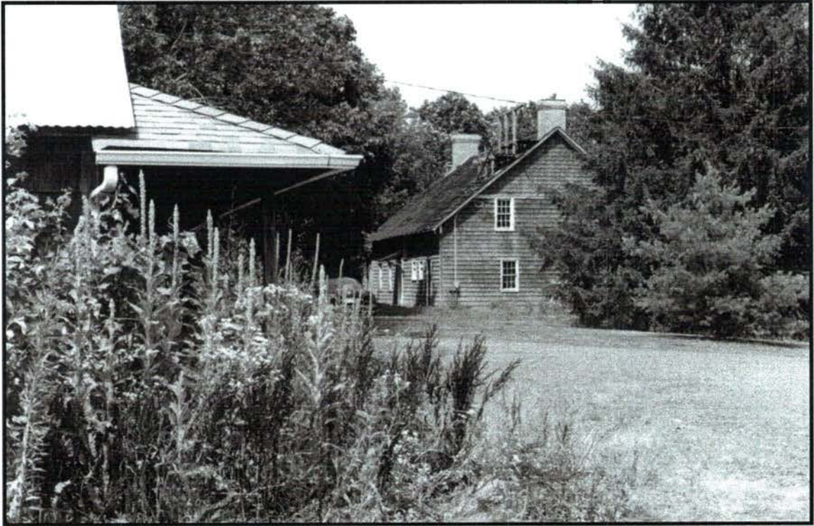
View of carriage barn and house, looking north. This relationship between out-buildings and dwelling is typical of the Dutch-American farmstead.
