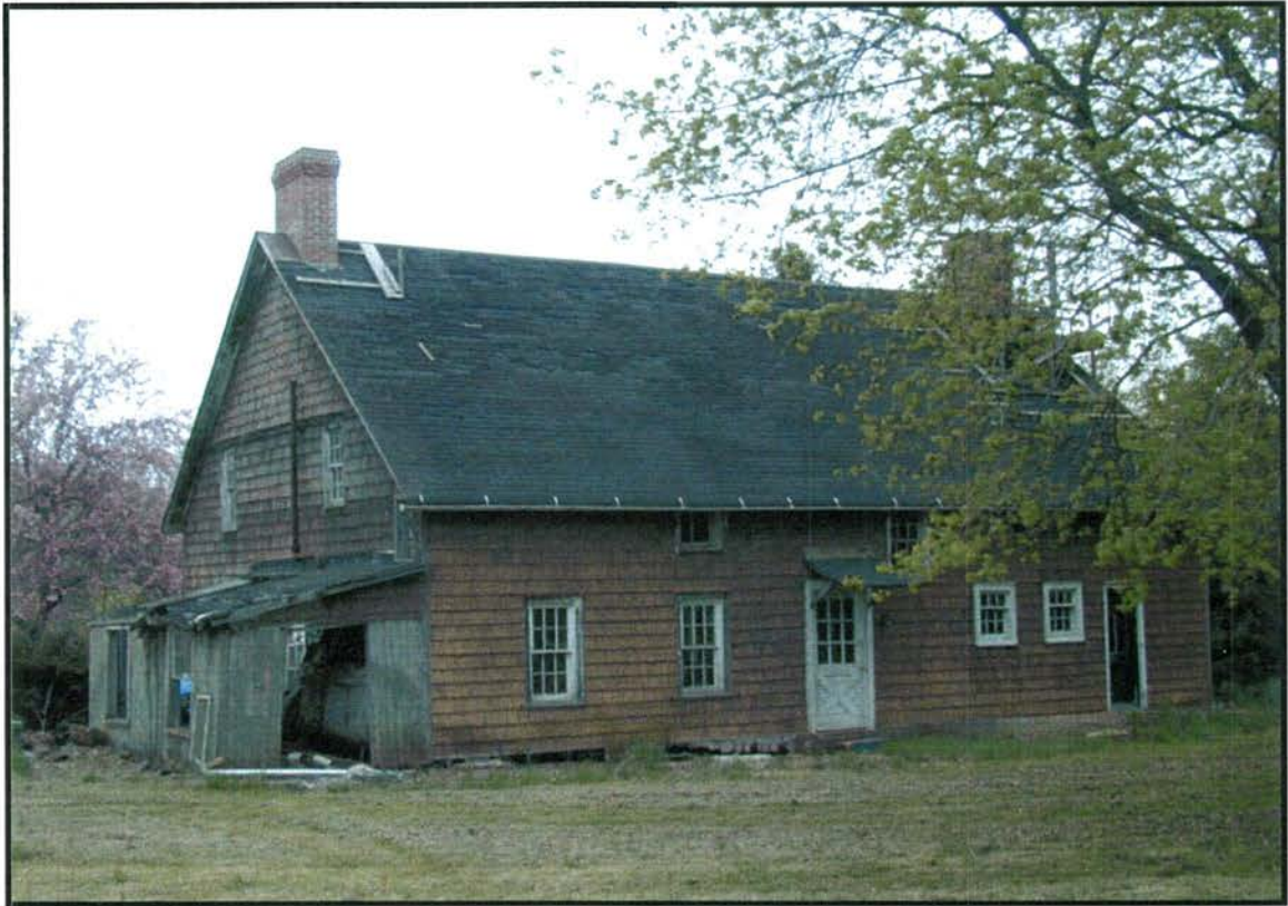
House from the northwest, showing lean-to addition that was removed during the study period.
