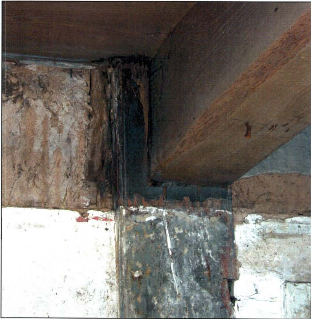
Room 100, detail of joint between the anchor beam and the post.
